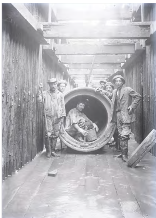
This photograph from the late nineteenth and early twentieth centuries shows workers building the sewers.
